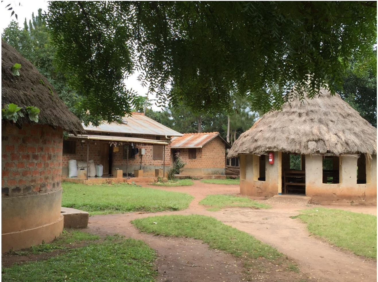
Buildings like these are in need of repair.
