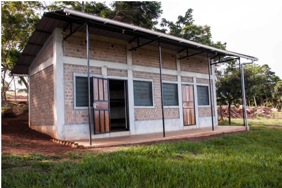
Newly constructed cabin at Musana Camps.
