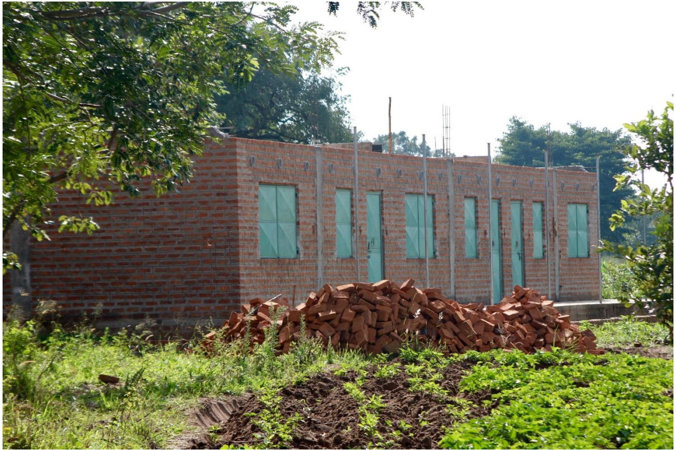
Our partly finished school at Kobwin Children's Center.
